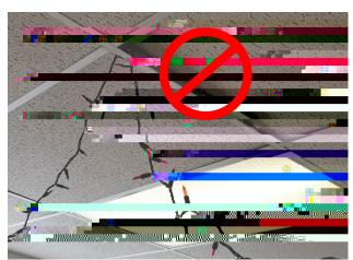
Do NOT drape wiring across T-bar framework. The stress from the weight of the ceiling tiles can cause breakage in the wiring, creating a hazard.
